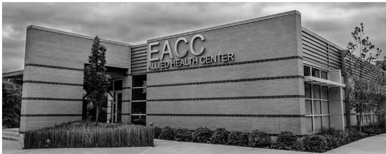
The Allied Health Center houses classrooms and labs for the health/science programs.
